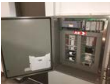
Georgia Pacific – Dudley, NC, USA Commissioned: March 2018
